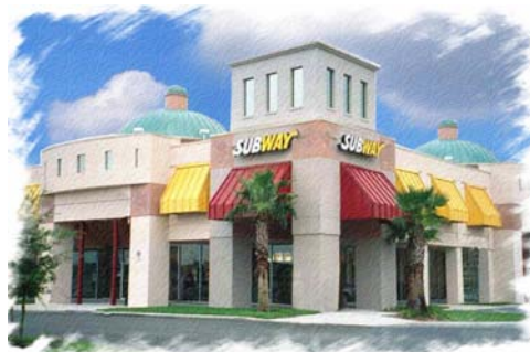
FRANCHISE SUBWAY® Orlando, Florida
